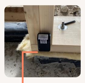
If the sensor will be exposed to rain, place the sensor upside down with the measuring pins closest to the ground.
